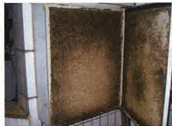
TV system panelboard filled with termite mud.
