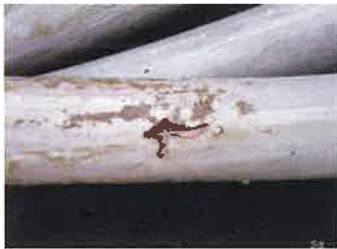
Trace of termite damage.
