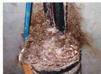
TV system panelboard filled with termite mud.
